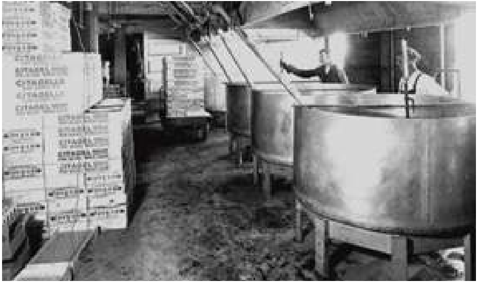
Figure 2: Jacketed steam kettles alongside stacks of block sugar at the Citadelle Cooperative plant in Plessisville, Québec.
