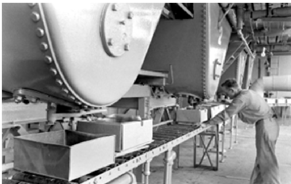
Figure 1: Pouring thickened super-heated maple syrup into block sugar molds at the Cary Maple Sugar Company plant in the 1930s.
