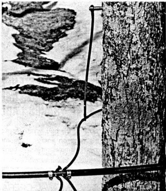
Figure 1. The sap collection networks were constructed of 5/16 inch plastic tubing as unvented, aerial-line systems with droplines at least 18 inches long. The small lateral lines were connected to 1/2 inch main lines.
