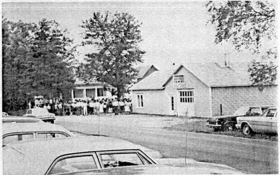
Gerald Lyndaker's modern sugarhouse near Belfort, N.Y. Gerald is installing an entirely new outfit consisting of two oil fired flue pans and a steam heated finishing pan powered by a 20 H.P. boiler.
